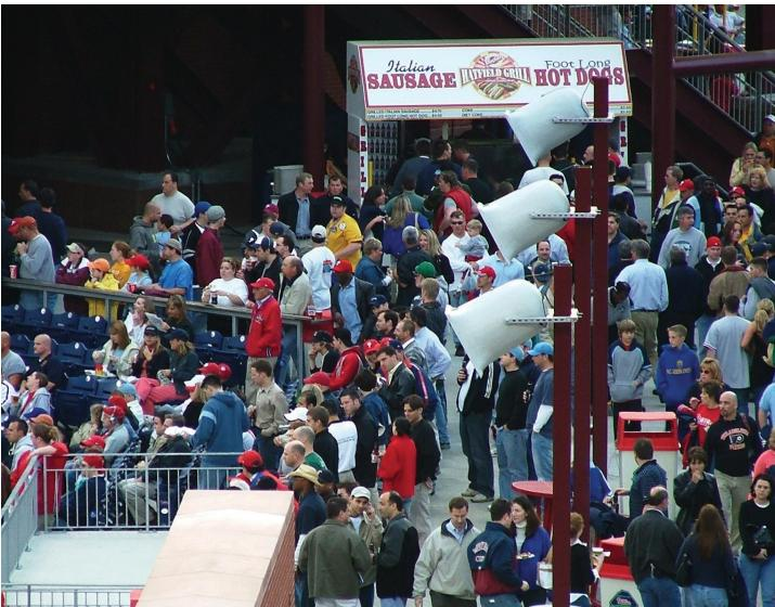
Day explained how both the architect, Ewing Cole, Philadelphia, PA and owner wanted a system that would have a long life expectancy and not deteriorate during the offseason. Philadelphia has rough winters, so the loudspeakers needed the capability to withstand cold inclement weather.
